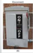
(B) Disconnect - An electrical device designed to interrupt the flow of electricity to a specific piece of equipment or a specific area of a building and/or unit. While inspecting electrical equipment the inspector will not touch or move the "cut-off" handle.
